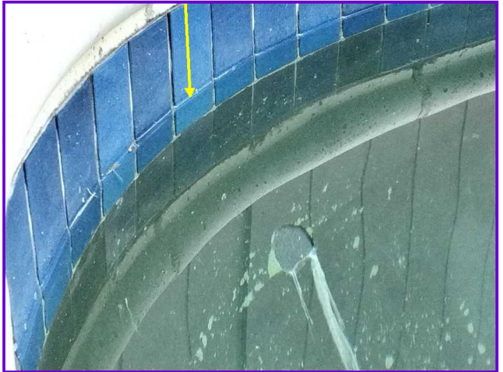
COMMENTS: The pool appeared to be reasonably level, as was evident from the water line on the tiles.
