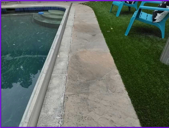
COMMENTS: The majority of the decking and coping appeared functional at the time of the inspection.
