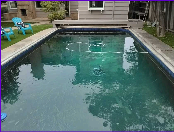
COMMENTS: The pool appeared to be reasonably level, as was evident from the water line on the tiles.
