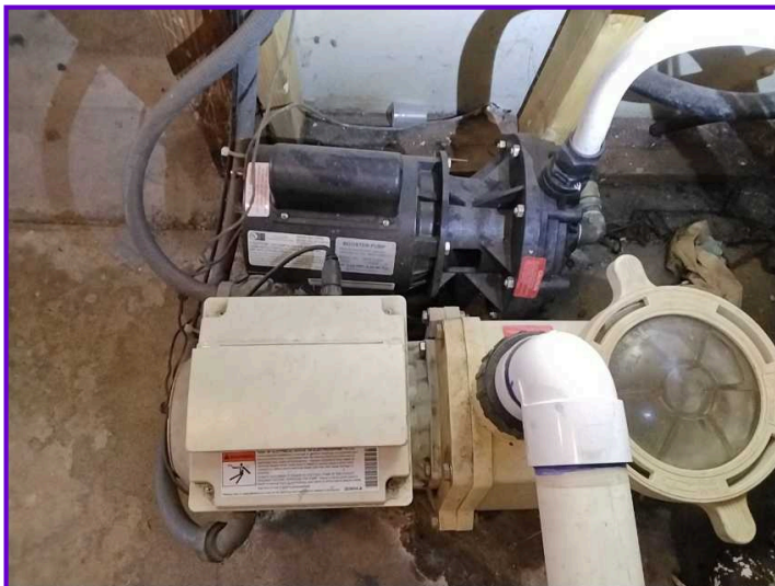
COMMENTS: The pool motors were operational and properly bonded for safety.
