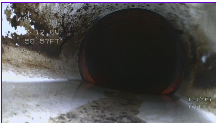
COMMENTS: At approximately 51 feet from the entrance, the sewer lateral drain line transitions to vitrified clay.
