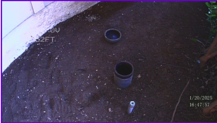
COMMENTS: The sewer lateral access is constructed of cast iron.
