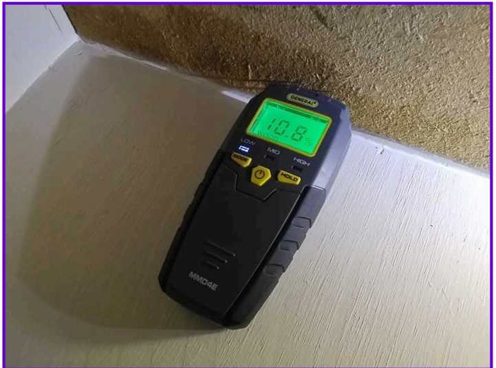
DEFERRED: During the inspection, moisture content was tested and found not to be a concern at this time.
