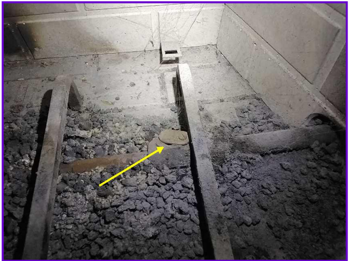
COMMENTS: The gas log starter in the fireplace appeared functional.
