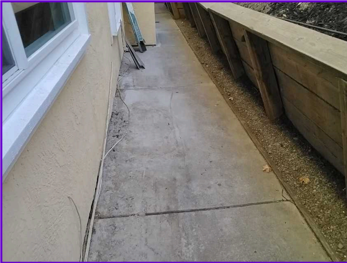
COMMENTS: The walkways at various locations around the residence are functional.
