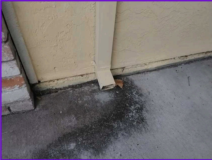
COMMENTS: The downspouts appeared to be clear and in satisfactory condition.
