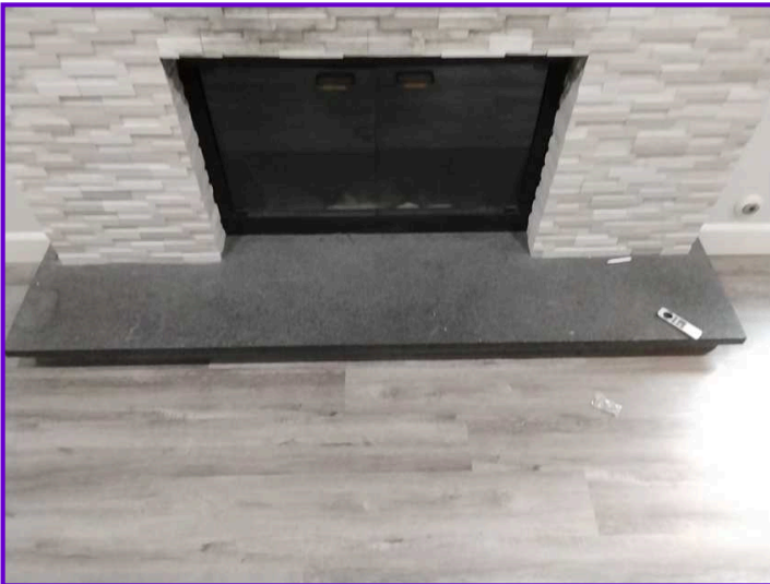
COMMENTS: The hearth extension is in satisfactory condition.
