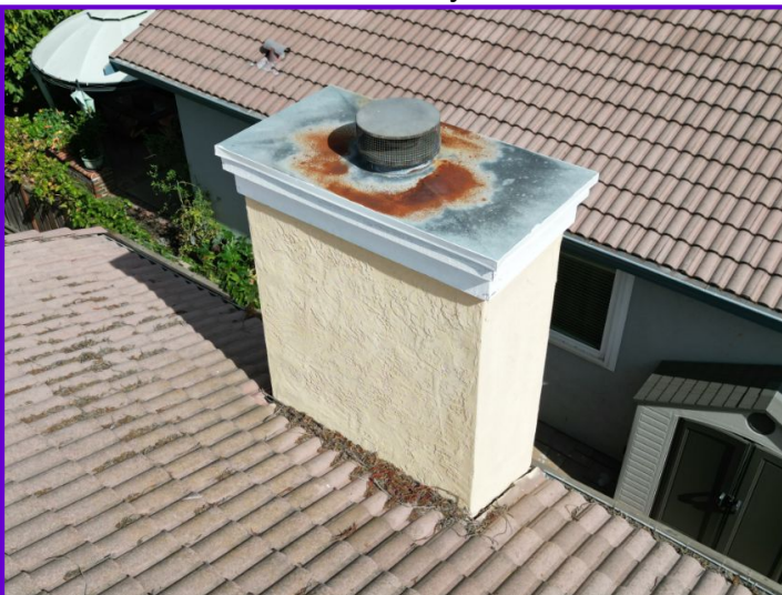
COMMENTS: The chimney structures had no visible defects.
