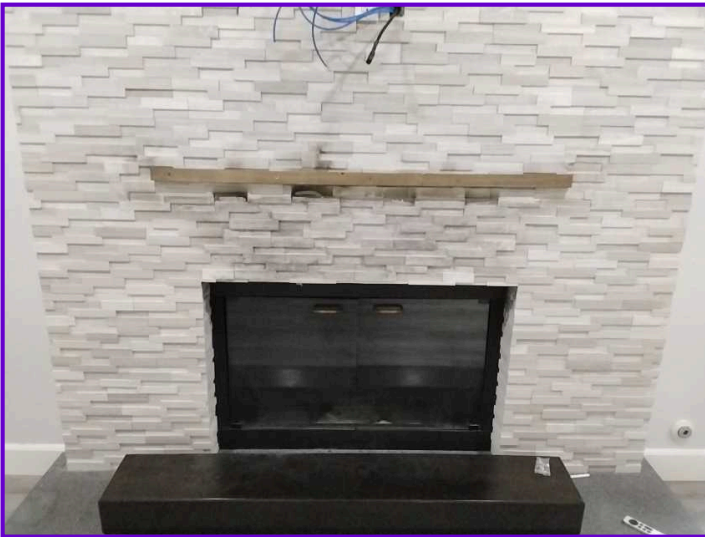
COMMENTS: The mantel and legs are in satisfactory condition.
