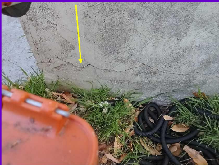
PREVENTIVE: There horizontal cracks in the stucco along the base of the walls.
