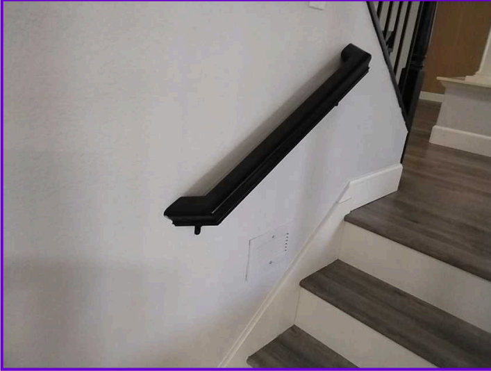
COMMENTS: The handrails appear to be functional and secure.
