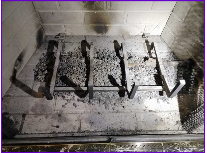
COMMENTS: The log grate appeared functional.
