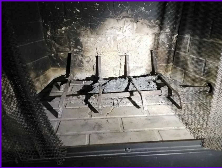
COMMENTS: The log grate appeared functional.
