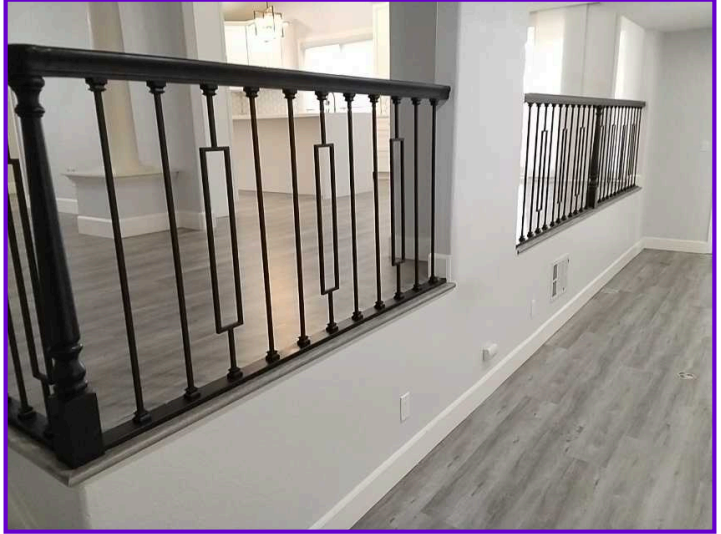
COMMENTS: The balusters rails appear to be functional and secure.
