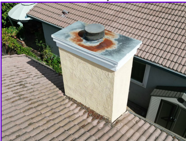
COMMENTS: The chimney structures had no visible defects.
