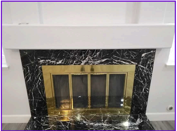
COMMENTS: The mantel and legs are in satisfactory condition.
